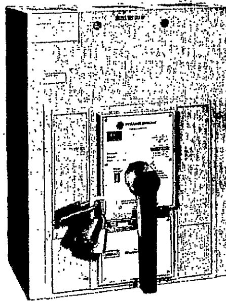
Fig. 3 Device Shown with Breaker Locked Open
