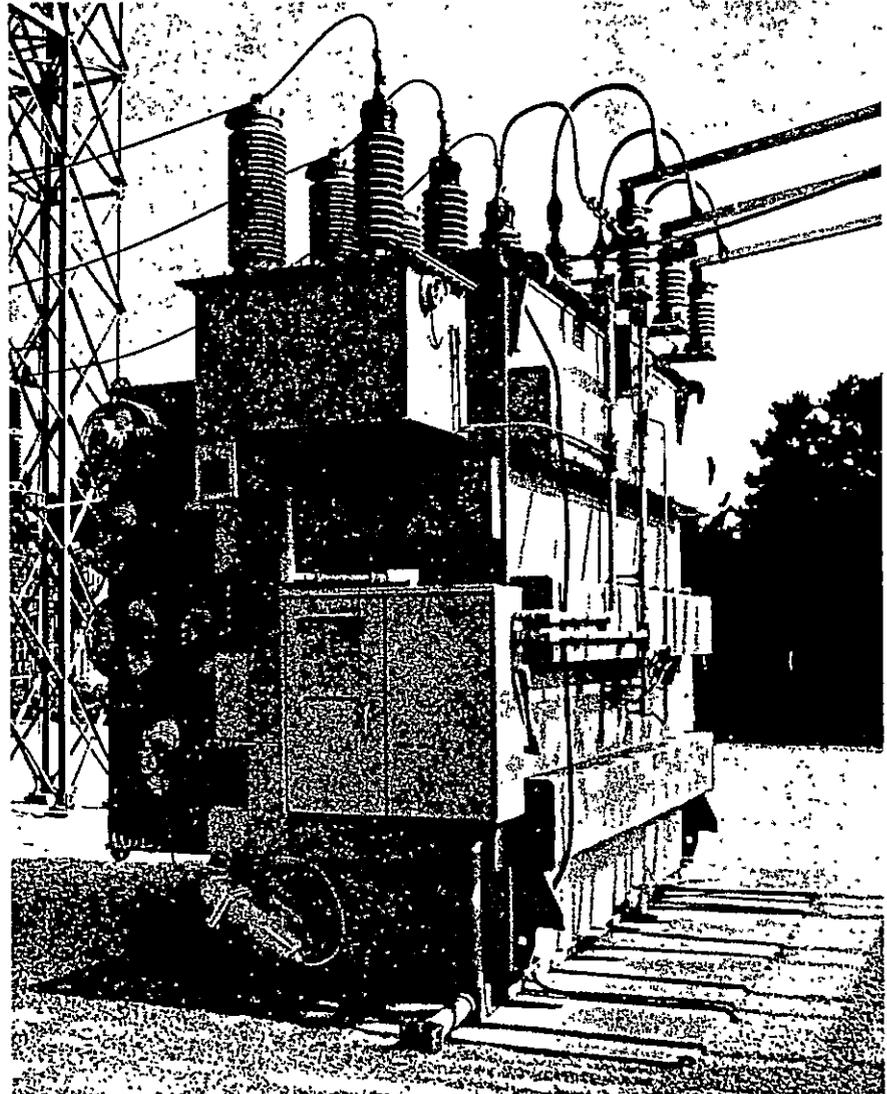
*Fig. 1. Load-tap-changing equipment, type LRT-200*
