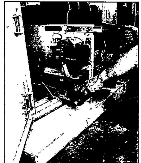
**6** Part way out the contactor will relatch in a "detent" position. To remove the contactor, press the latch bar down and at the same time pull the contactor forward. Lower the contactor to the floor and roll out of the way. (The contactor weighs approx. 125 lbs.)
