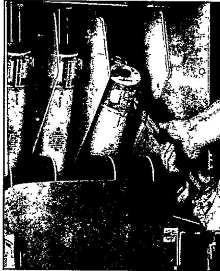
**2** Remove three main fuses (B) using the fuse puller (K) supplied. See operating instructions (C) inside medium-voltage door.
