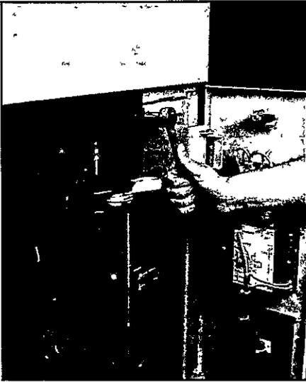
7 To remove the Isolating Switch (H), remove two bolts as shown.
