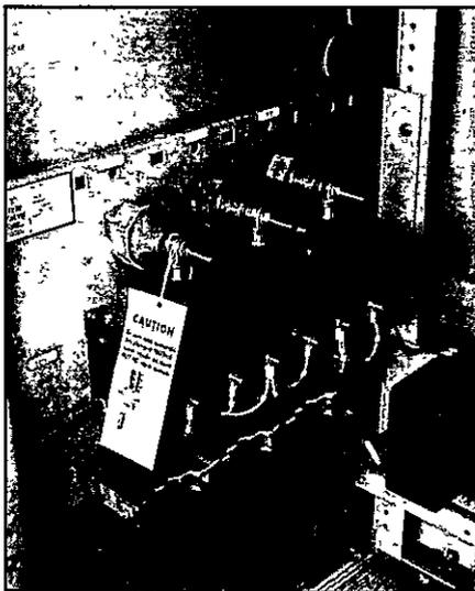
10 Refer to load cable instruction tag (J) located in starter at motor terminal for load wiring instructions.
