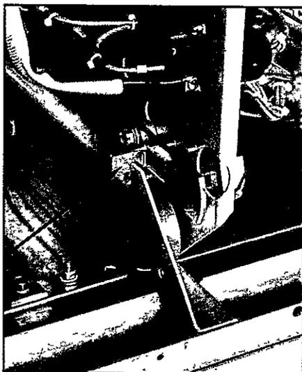
**13** Return contactor to its compartment and make sure detent latch is engaged.
