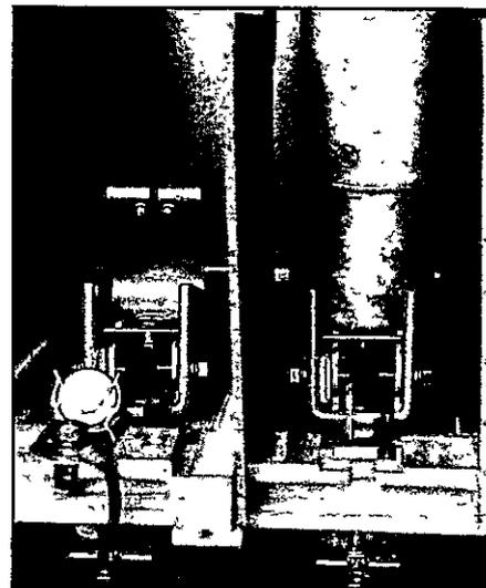
**15** Install the three main power fuses. Make sure fuse is fully seated on bottom fuse holder located on the contactor.
