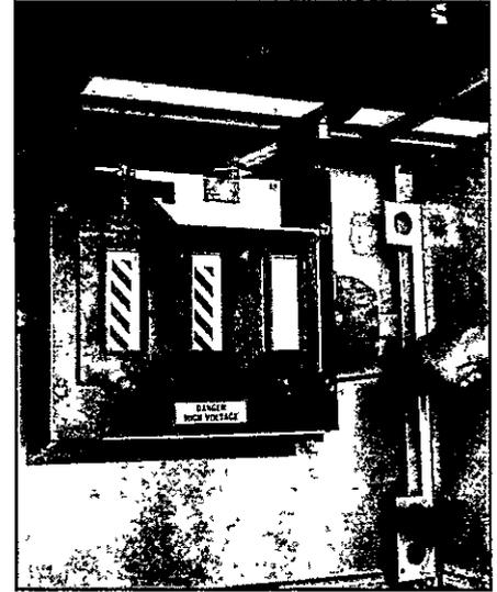
9 If cable is used to connect the line stabs, loosen four pan head screws approximately three turns. Lift rear barrier and shutter assembly up and off the screws. Disconnect the shutter drive lever using the keyhole in the lever. Starter is now ready to wire.
