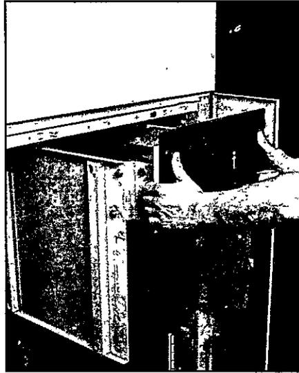
8 Pull Isolating Switch forward. **Caution:** It has no latch and will pull completely out. However, it weighs only 75 lbs. and can usually be handled without a crane or lift.
