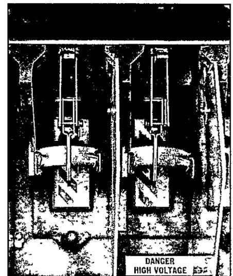
11 After wiring, reverse the procedure to reassemble. Slide Isolating Switch in place and secure with two bolts. Refer to Steps 7 and 8.
