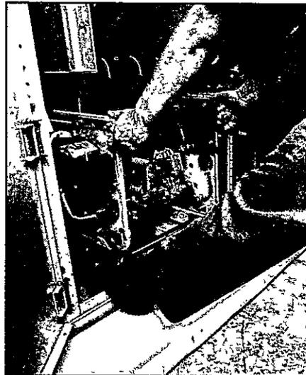
**5** To remove contactor (E), lift latch (G) on bottom left-hand corner of contactor and at the same time give the contactor a sharp pull forward.
