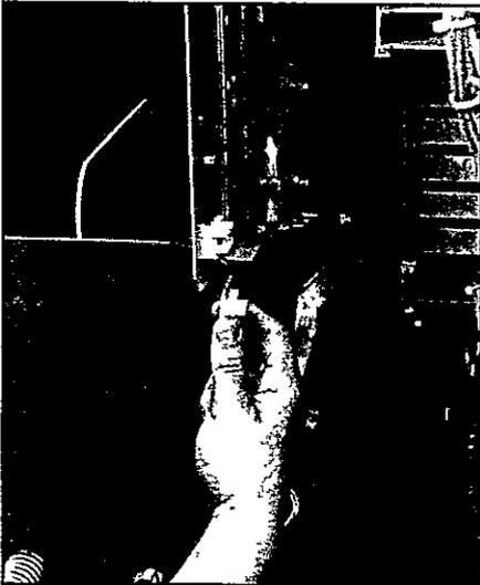
**4** Disconnect the auxiliary interlock terminal block (F) on the Isolating Switch.
