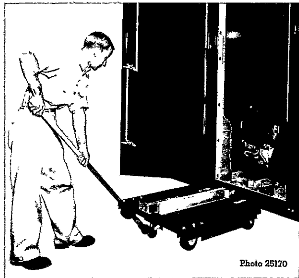
Fig. 2. The dolly is maneuvered into position by means of a fifth wheel device, as shown. The circuit breaker compartment door must be fully open. To insure proper vertical alignment of the dolly with the gear, raise or lower dolly as required, by means of leveling bolts (See Fig. 1)
